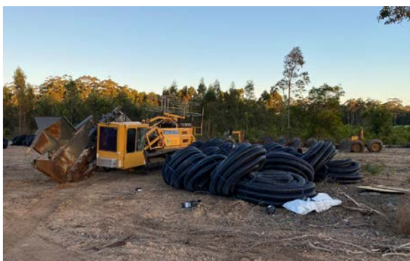
Stage 2 Ripping completed (above) and drainage equipment and aggregate mobilised to site in accordance with the subsurface drainage timetable (below)
