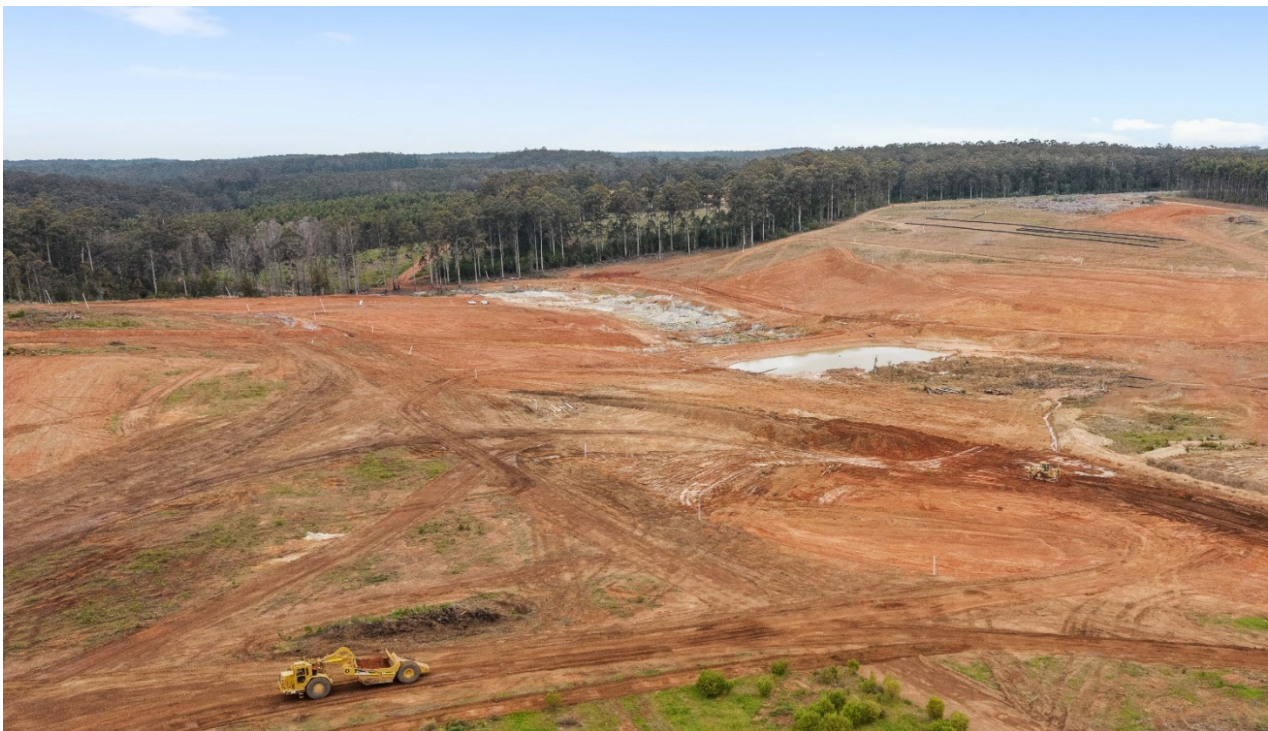
Dam site progresses under landowner construction
